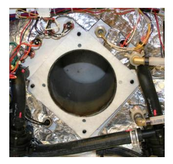
3. Remove the Mounting Gasket from the boiler tank's front plate and the Propane-Burner.
