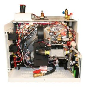
2. Carefully lift the Propane-Burner away from the Aqua-Hot.
