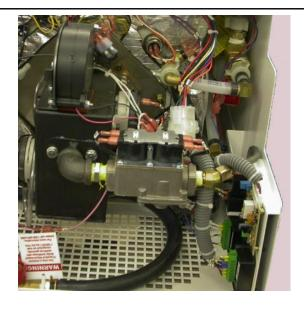
2. Using an 11/16 wrench, loosen the nut securing the fuel line to the gas valve assembly.
